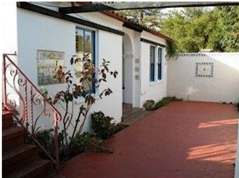
Figure 6. Photograph showing 766 Santa Ynez Street (Redfin, 2022).
