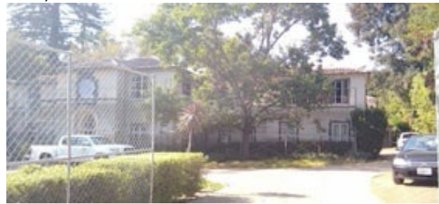
Figure 10. Photograph showing Mediterranean-style house at 678 Mirada Avenue (Environmental Science Associates, San Juan Residential District Historic Survey , 2021).
